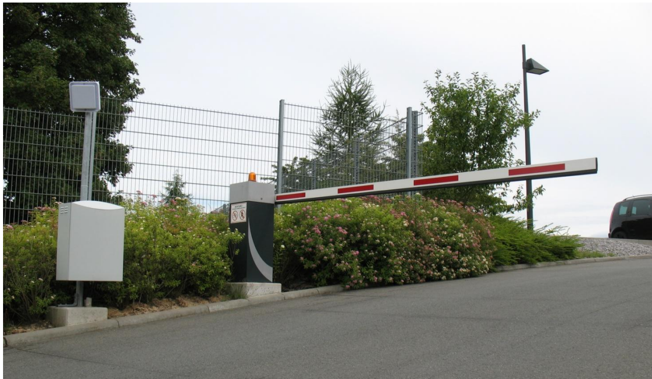
Figure 18: Positioning of the antenna
